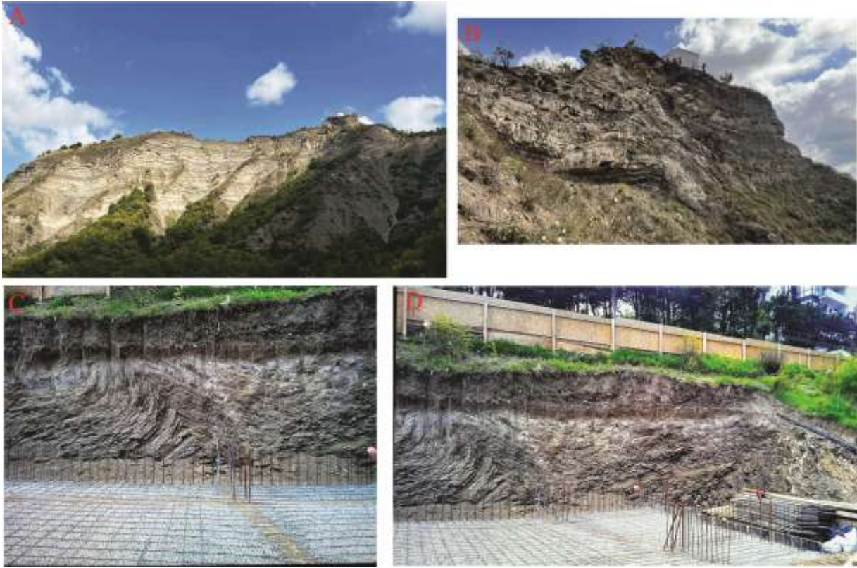
Fig. 2. Secondary structures in the river Vere valley.
