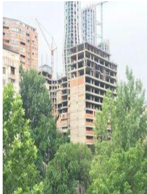
Fig. 1. An unfinished house
