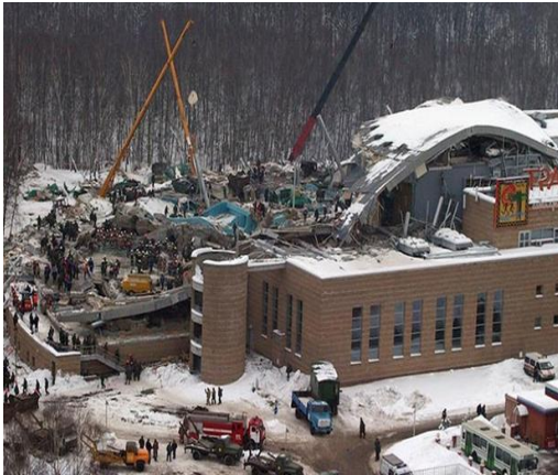
Fig. 8. "Transvaal" roof accident
