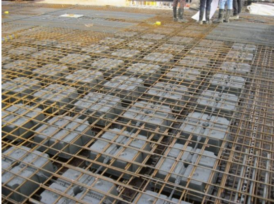
Fig. 3. U-BOOT BETON system
