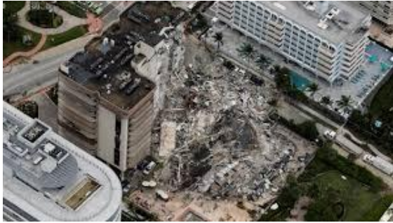
Fig. 6. Wing collapse in Miami
