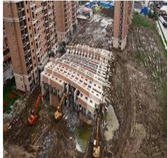
Fig. 1. A collapsed house in Shanghai
