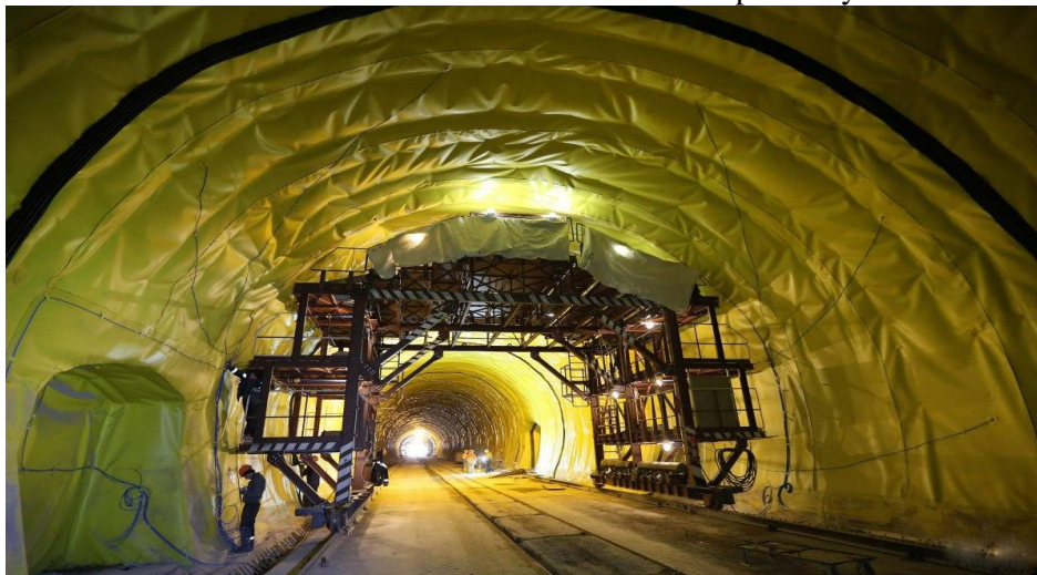
Fig.2.Tunnel waterproofing with polymeric membrane
