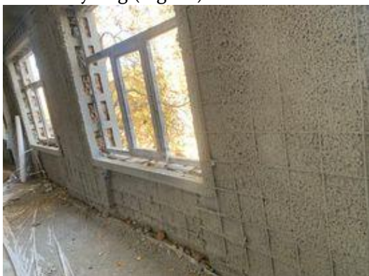
Fig. 11. Torcreting stage II
