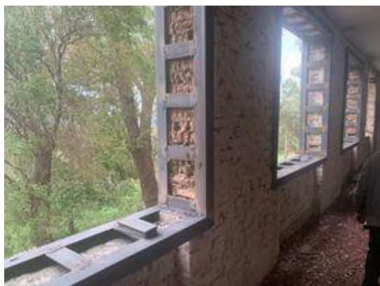
Fig. 1. Reinforcement of window openings
