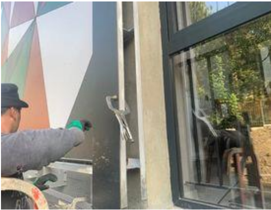
Fig. 10. Arranging the frame of the panel
