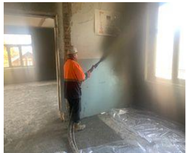
Fig. 9. Torcreting process
