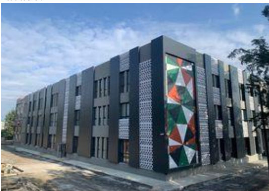
Fig. 12. The left panel of the main facade
