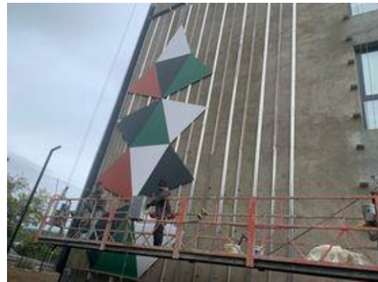
Fig. 7. Installation of the panel vertically
