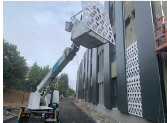
Fig. 3. Installation of figured white panels
