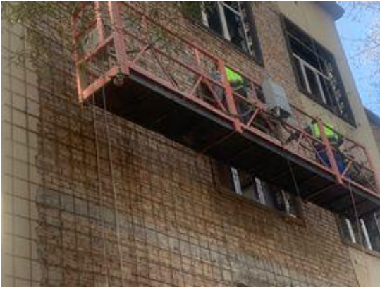
Fig. 5. Installation of nets with a hanging basket
