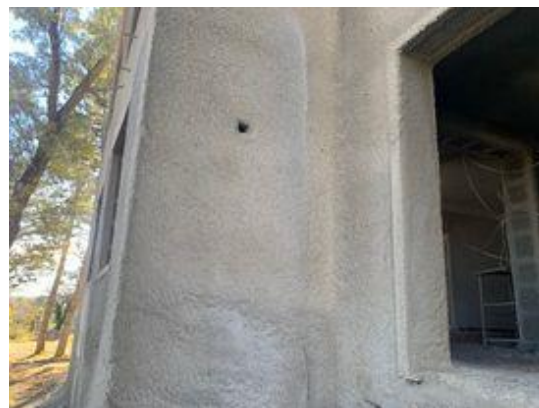
Fig. 13. Outer surface of the wall
