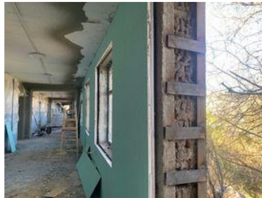
Fig. 14. Plasterboard on the inner wall
