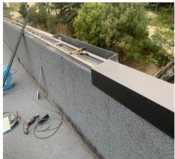
Fig. 15. A box of wall panels
