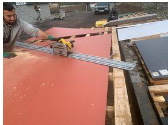
Fig. 4. The process of cutting the wall panel
