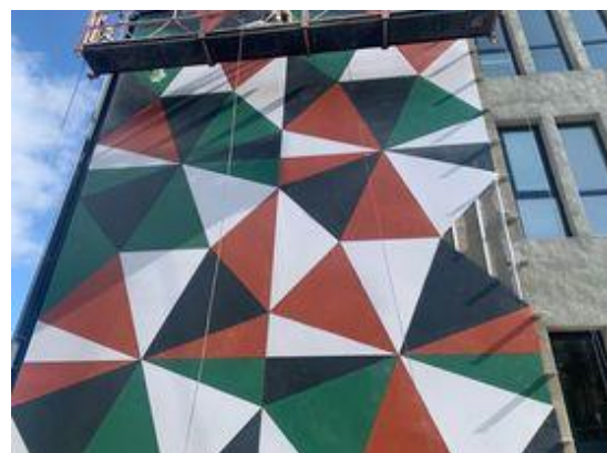
Fig. 9. Installation of the second part of the panel
