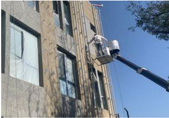
Fig. 1. Installation of aluminum brackets and beams
