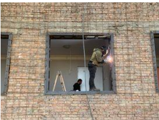
Fig. 7. Weld the grid to the corner
