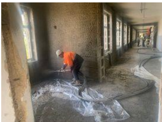
Fig. 12. Torcreting stage III
