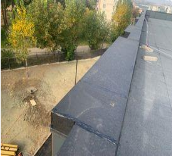
Fig. 16. Covering wall panels with tin
