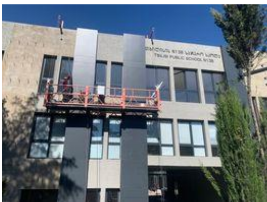
Fig. 2. Installation of main wall panels
