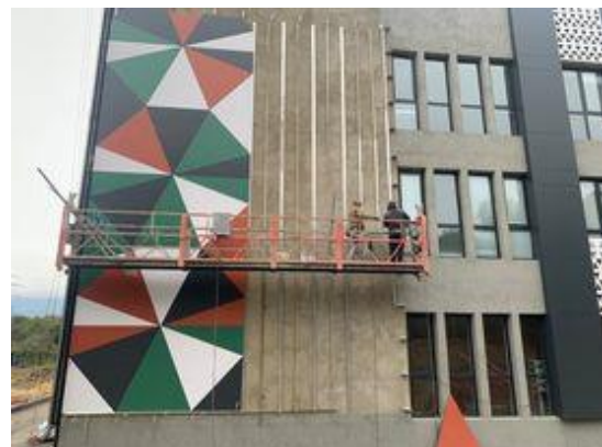
Fig. 8. Completed first part
