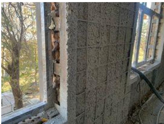
Fig. 10. Torcreting stage I
