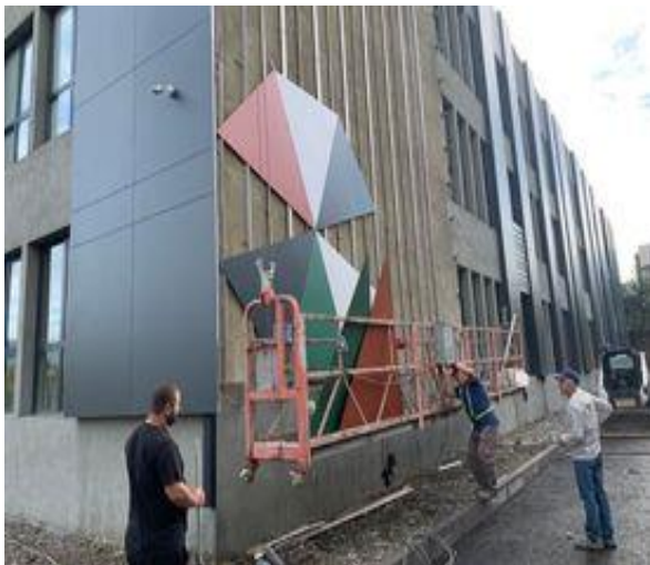
Fig. 5. Start panel installation
