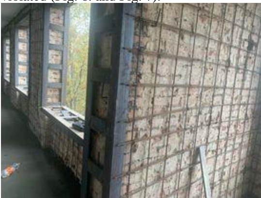
Fig. 6. Mesh on the inner surface of the wall
