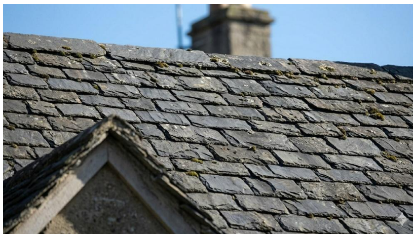
Figure 6. Clay shale roofing
