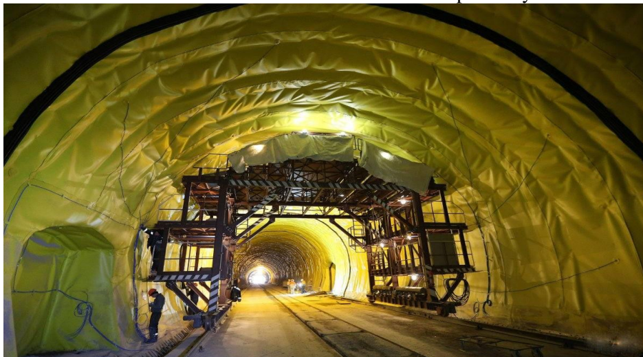
Fig.2.Tunnel waterproofing with polymeric membrane
