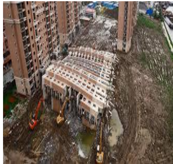
Fig. 1. A collapsed house in Shanghai
