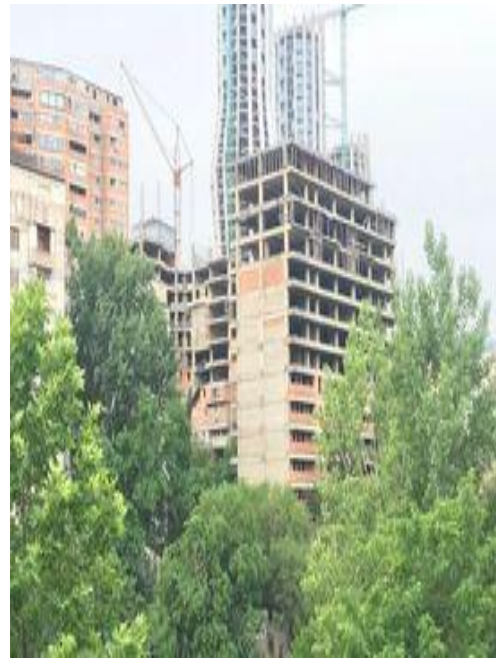
Fig. 1. An unfinished house
