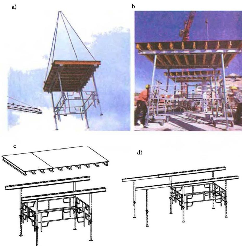
Fig. 4. „RASCHAL“ "stellMAX" mold with folding frame: A - mold transportation by crane; b - moving the mold with a cart c - installation and dismantling of the platform; d – mold Extension of the table
