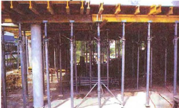
Fig. 1. „PASCHAL DEK“ roof formwork systems
