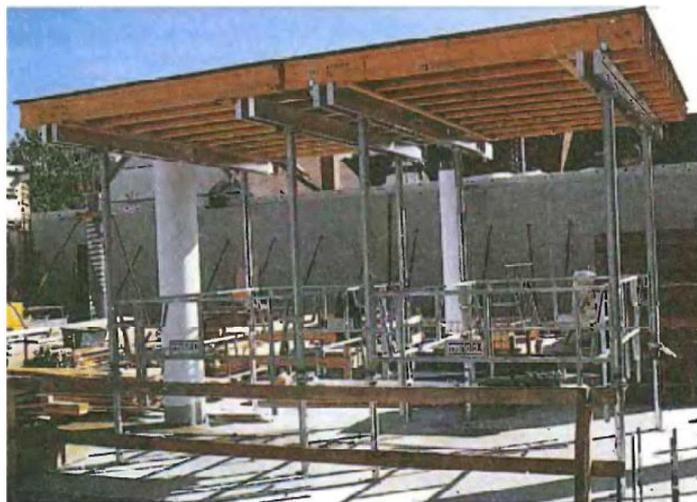
Fig 3. „RASCHAL“ A view of the folding frame mold
