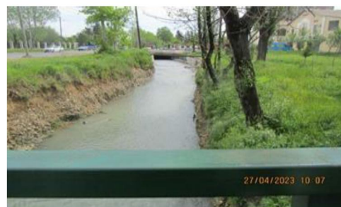
Fig. 4. View of the River Oghaskura upstream, from the metal bridge, to the point of outflow from the artificial bed
