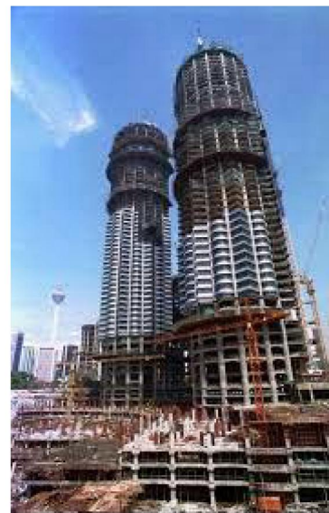
Fig. 7. Tower construction process
