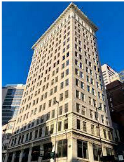
Fig. 1. The world's first concrete skyscraper "Ingalls Building", built in 1903 in Cincinnati (USA), a 16-story, 64-meter-high building, is considered to be the world's first skyscraper built of reinforced concrete. Its construction, which lasted for 8 months, received a great response, because
