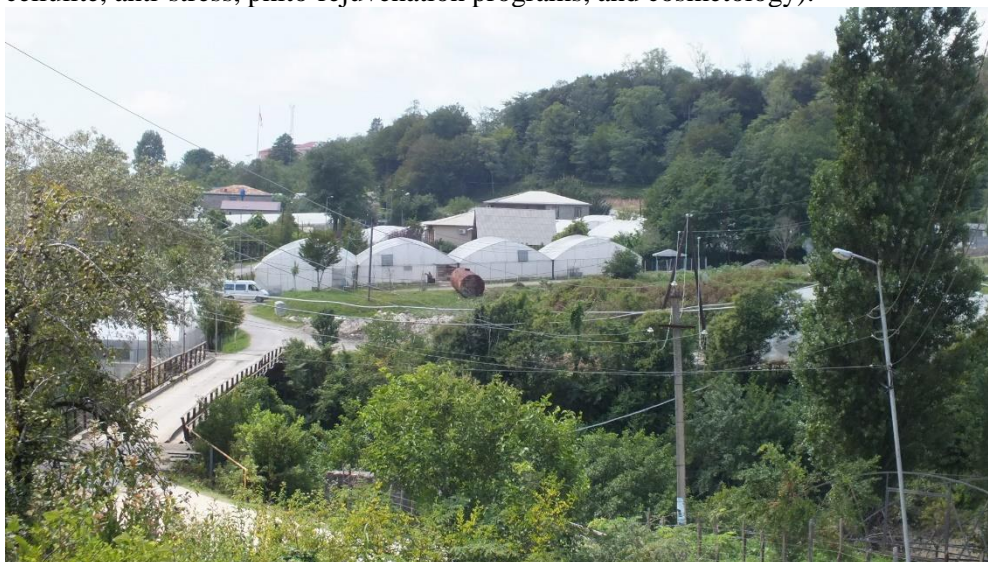
Fig. 3. Greenhouses in the resort Tsaishi, which utilize local thermal mineral waters (photo by M. Tutberidze).
